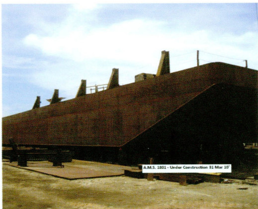
The A.M.S 1801 under construction in Darwin.
